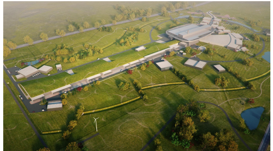
European Spallation Source (ESS), Lund, rakenteilla
