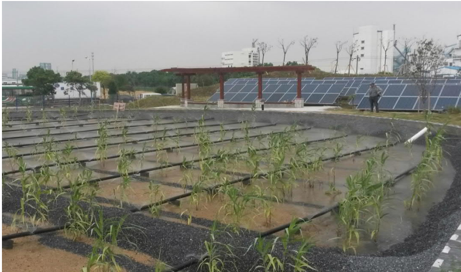
Continuous Vertical Flow Wetland, China
