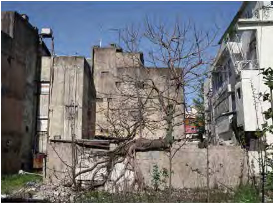
Plant at 84th Street, Jeonju, 2012.
