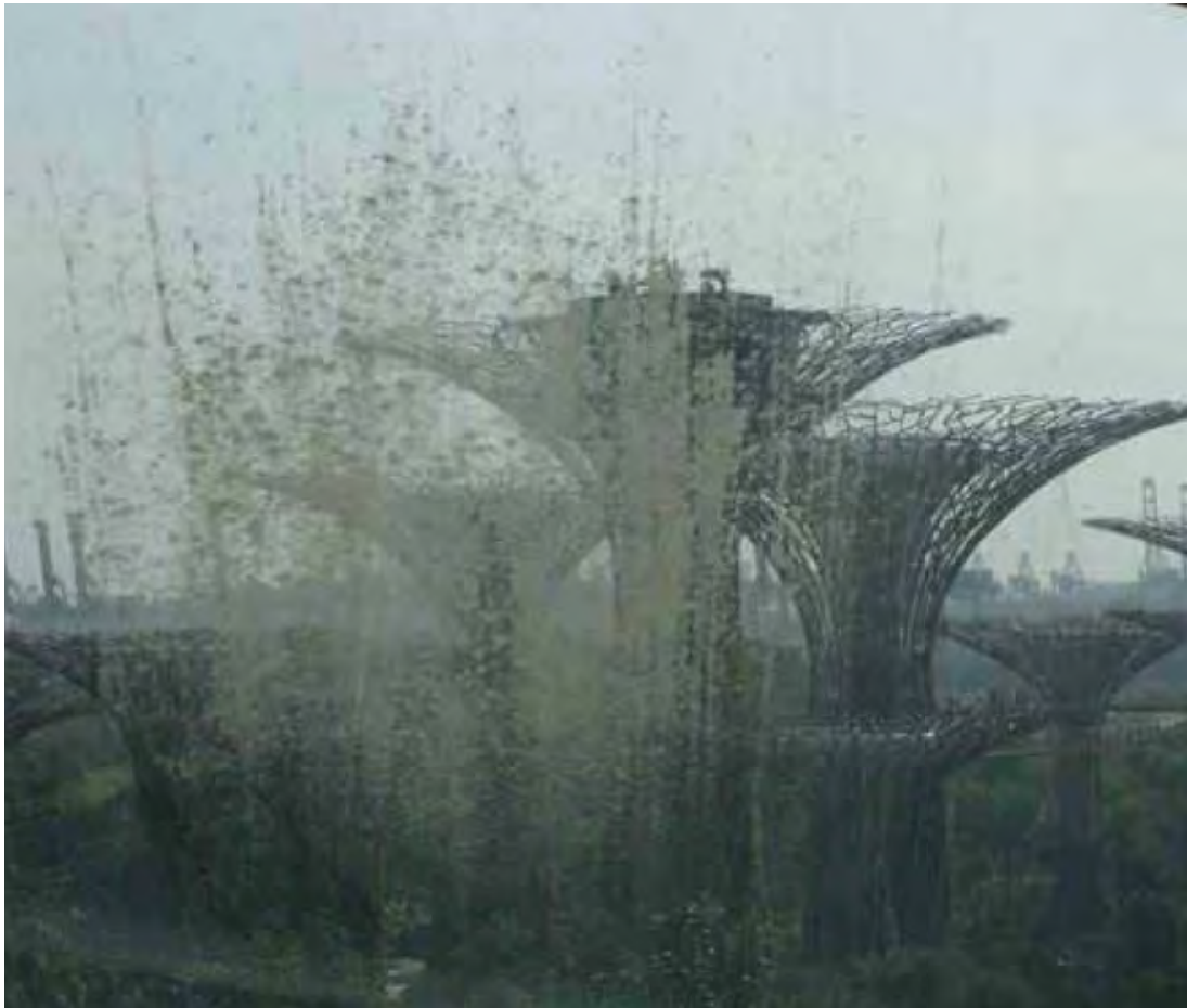
Fig. 12 While touring this perfectly maintained space, I am drawn to one pane of glass that reveals what happens when this space is not so meticulously maintained by so many labouring hands. This grungy smear blocks the view of what should be such a photogenic landscape, one that includes not only the Garden's Supertrees, but also an imposing sweep of port-land cranes, such potent markers of Singapore's booming economy. It is at this moment that the massive and impressive edifices of the conservatories suddenly appear more like fragile, thin envelopes enclosing a precariously simulated Eden. At the same time it becomes clear that it is the very conception and construction of this Earth Ship—the excessive extraction of plant species, metals, and materials—that is accelerating the destruction. I realize then that this is not just a garden of leisure and spectacle. It is both a living memorial to an already vanishing world, and a thriving fantasy of the earth's immanent undoing. It is the very materialization of this fantasy that is bringing on the end-of-times. Perhaps the only response is to write against this dream: to conjure another possible future. The question then becomes how to work athwart the apocalyptic future that this garden dreams so furtively? What other fantasies can be conjured?
