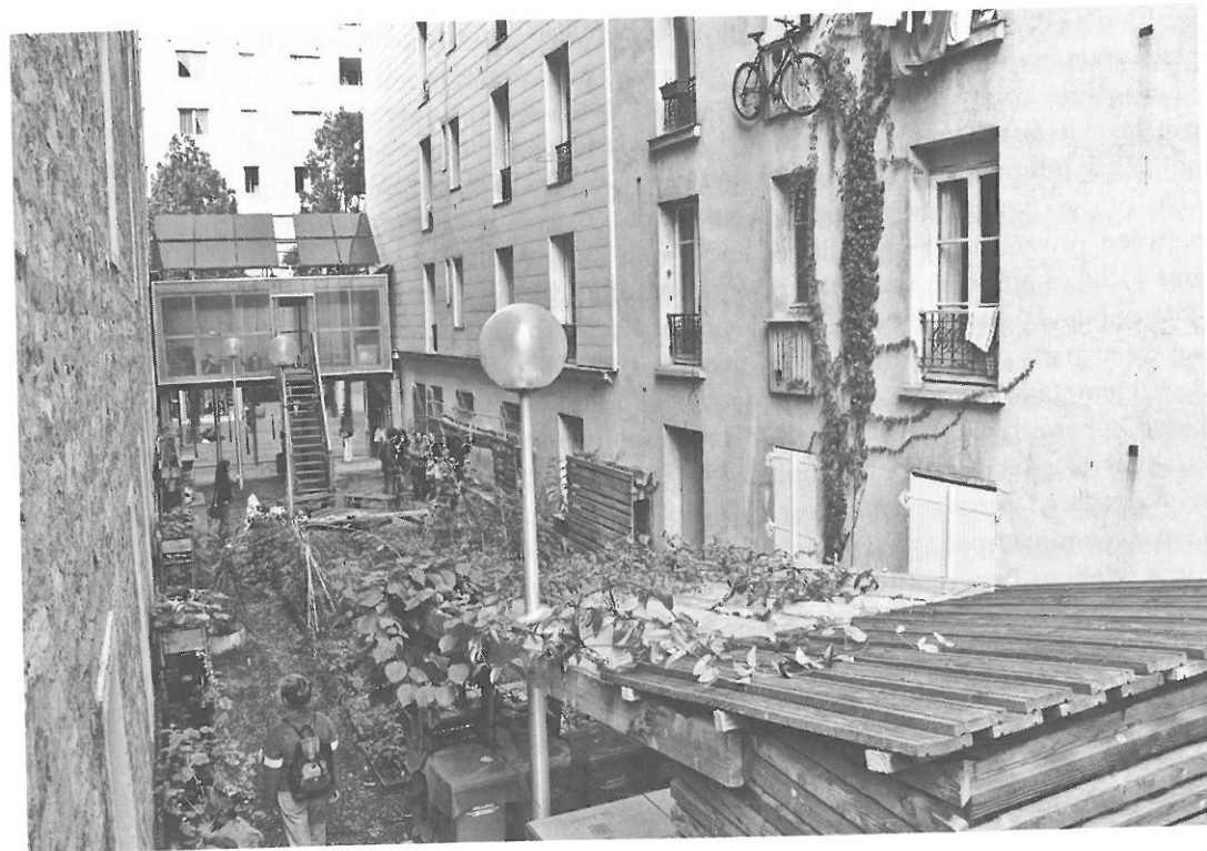
2.3 atelier d'architecture autogérée, Passage 56 , cultural and ecological space managed by residents of St. Blaise neighbourhood, Paris, (2005–ongoing). Photograph: Constantin Petcou (2009).
