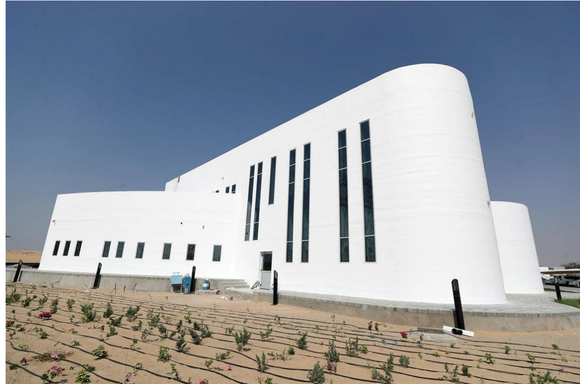
Eco-sustainable 3D printed house (local and recycled materials) - Tecla, 3D printed by WASP
